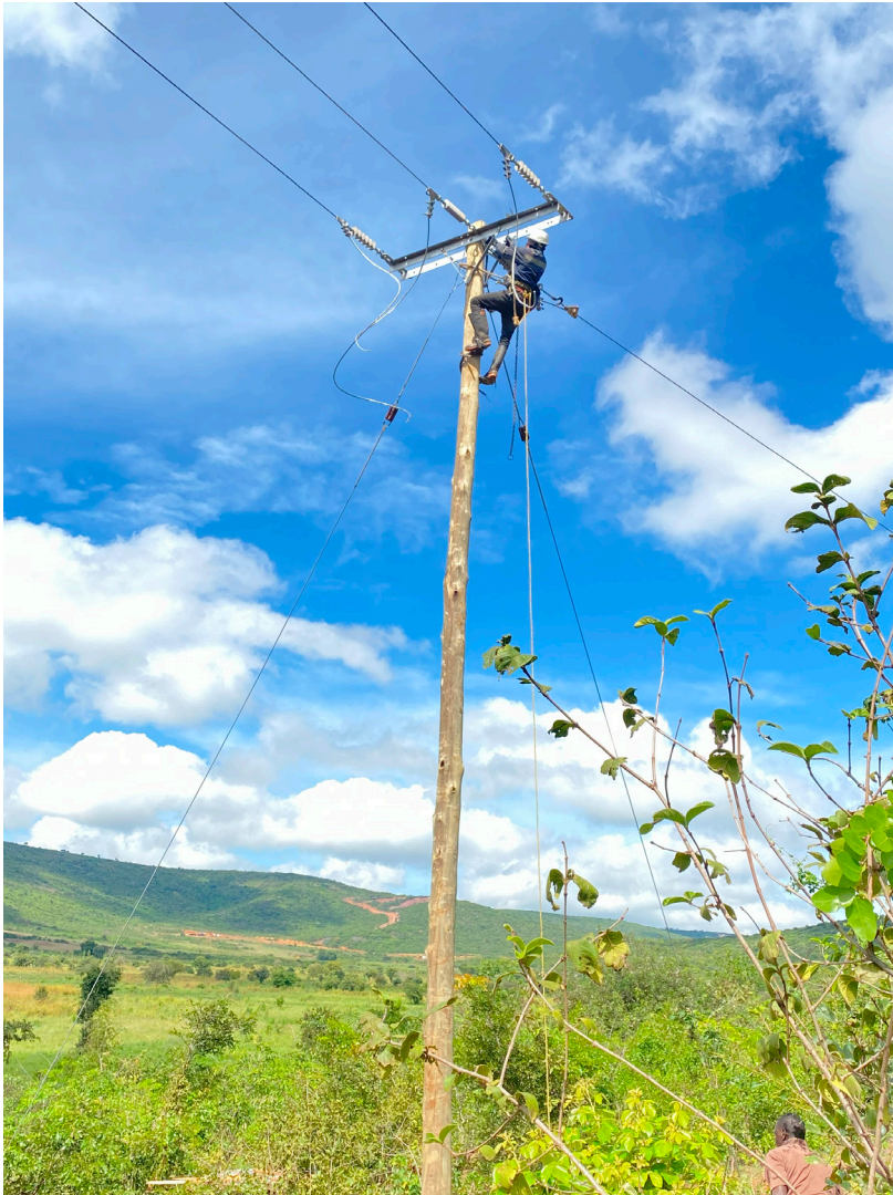
Extension Of 33kV Line R/L 3.54 KM and Establishment of 800kVA 33/0.4kV Transformer Substation at Nestory Makune's CIP (Mwazimba-Shinyanga)
