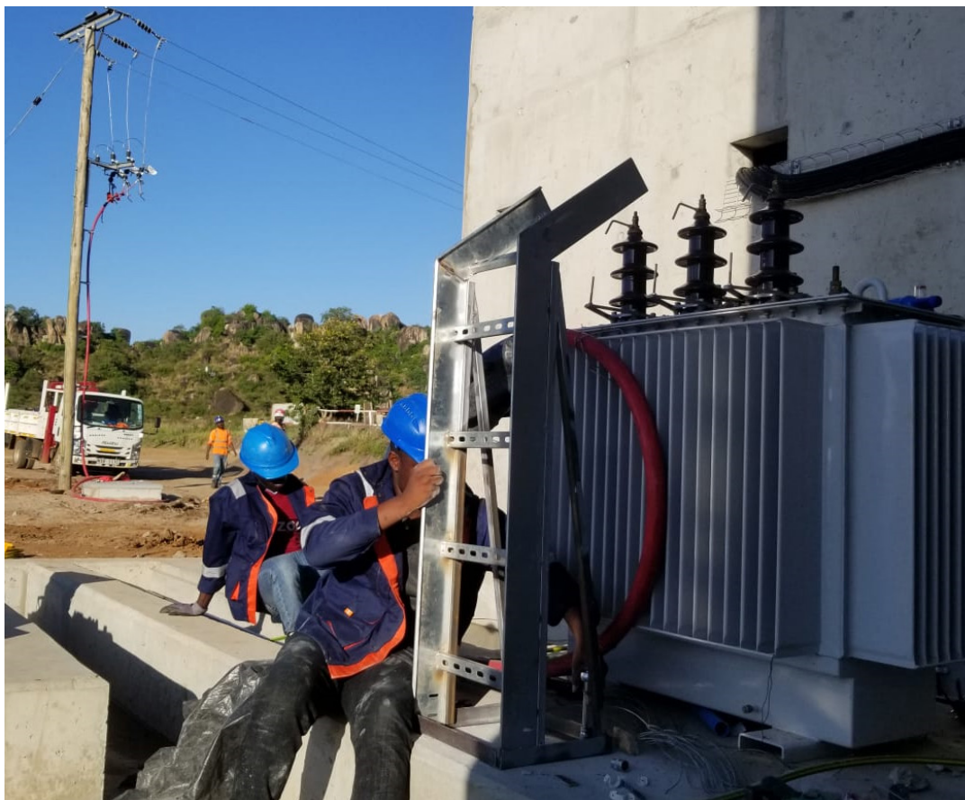
400kVA Transformer Installation
